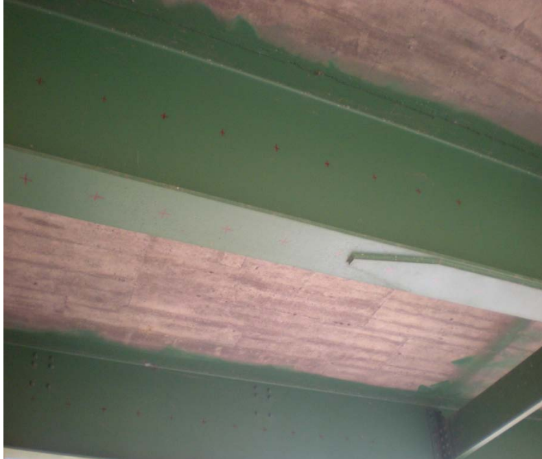
Figure 4.4 Markings at one foot intervals on the web and bottom flange of each beam
