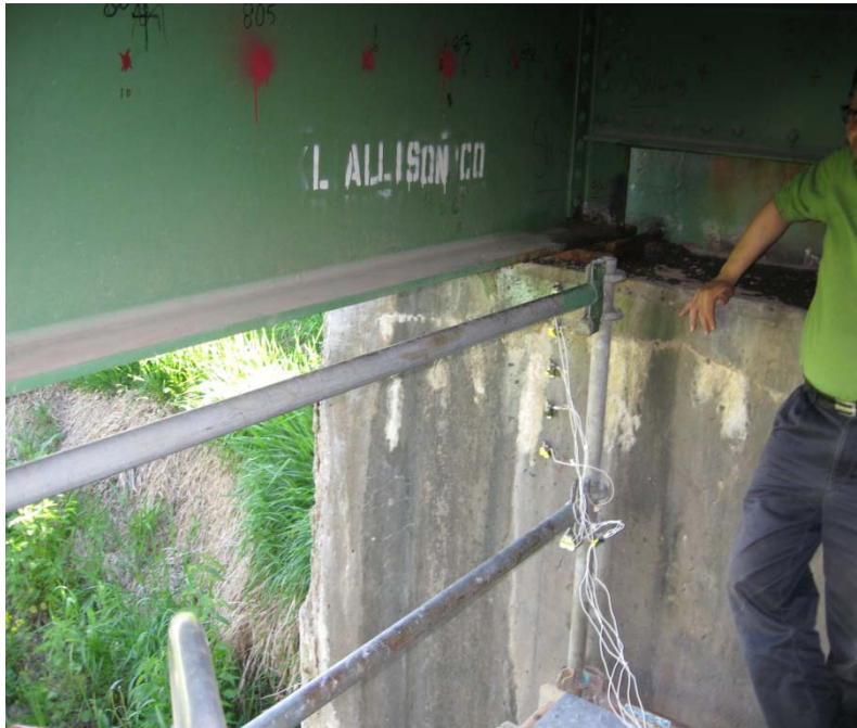
Figure 4.27 Operational vibration response measurement of a strip of the vertical face of an abutment
