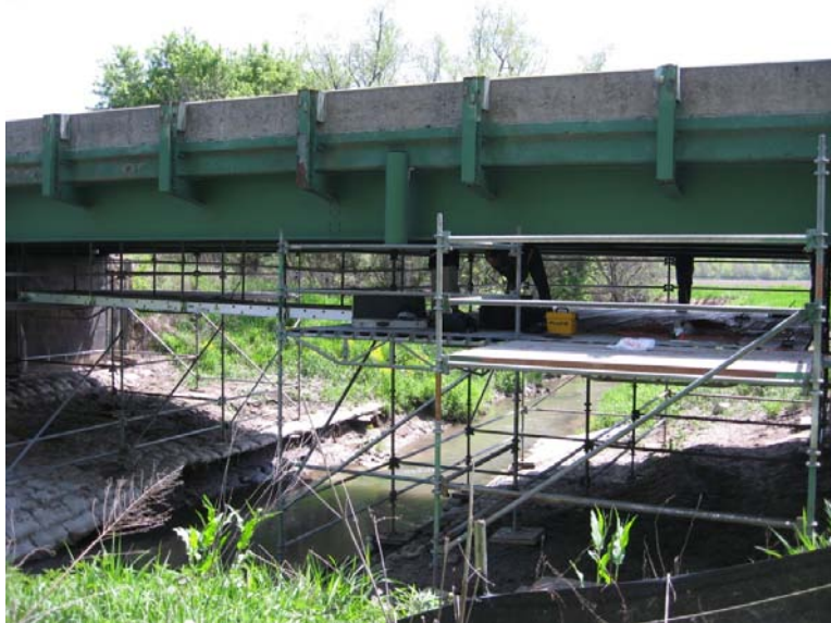
Figure 4.13 Scaffolding that provided access to the entire superstructure
