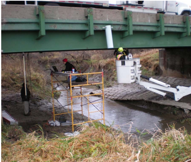
Figure 4.5 Single scaffolding tower used to impact beam 1 at node 12
