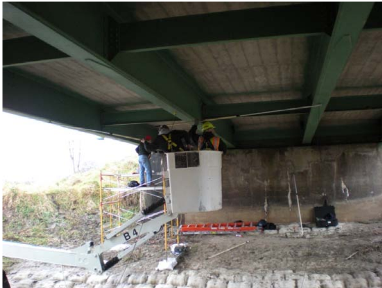
Figure 4.7 Snooper truck and long poles used to access the bottom flange of each beam
